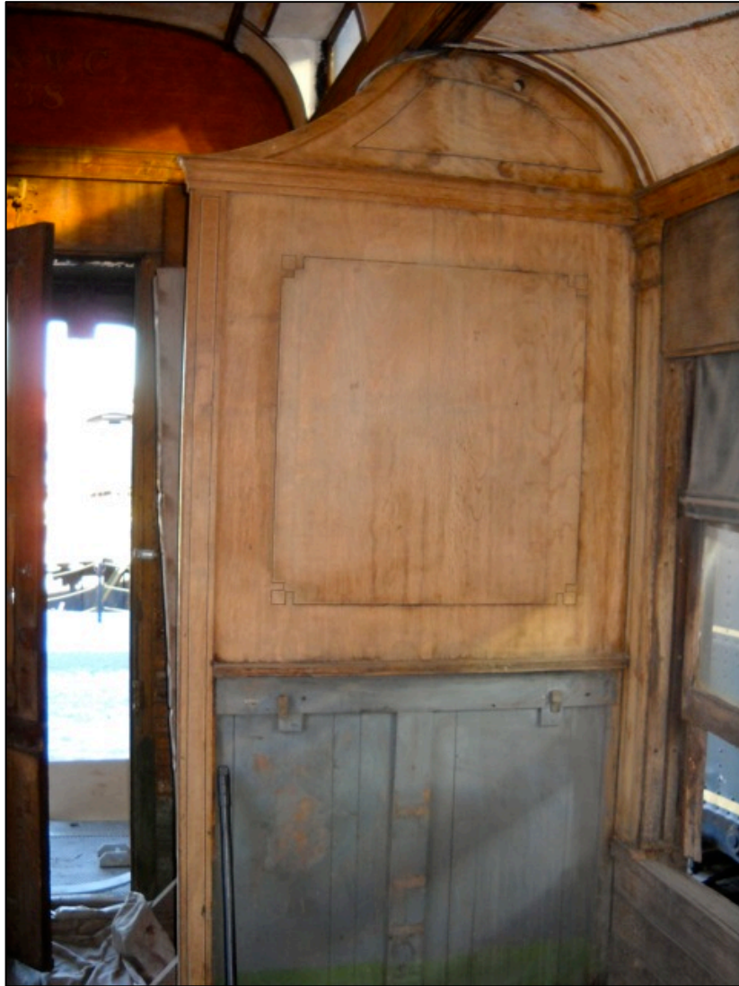
Panel after cleaning, before sanding.
